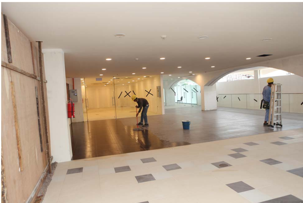
Works at the Open Café and Commercial areas are almost completed.
