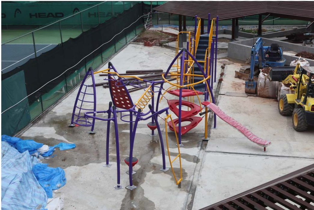
Playground equipment works are in progress.
