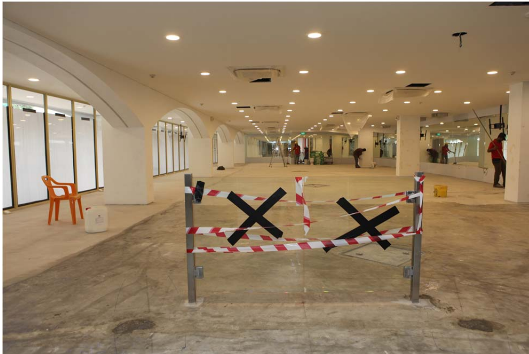
Ceiling and wall finishes at Gym area are completed.
